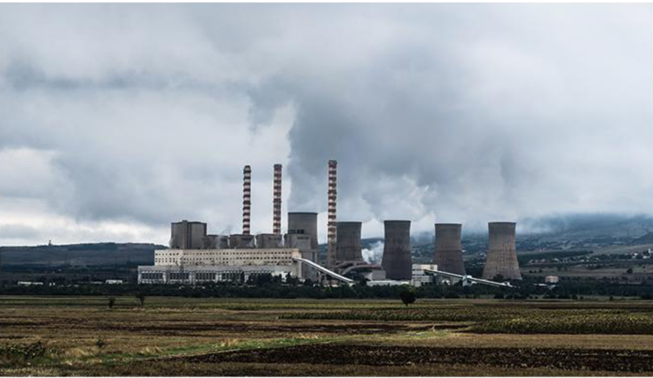
Flue gas desulfurization
