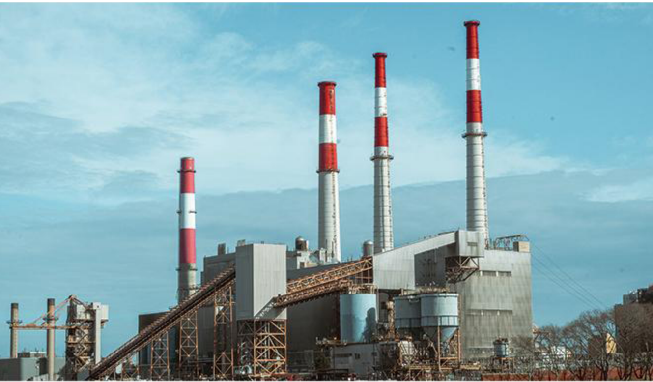
Cement thermal power
